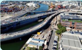
Entry and exit ramps at MacKenzie Road
