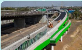
Hyde Street ramps
